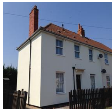
After Solid Wall insulation
