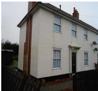
Before Solid Wall insulation
