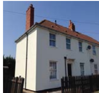
After Solid Wall insulation
