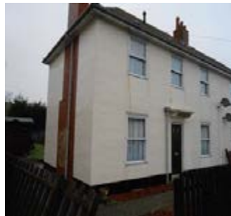
Before Solid Wall insulation
